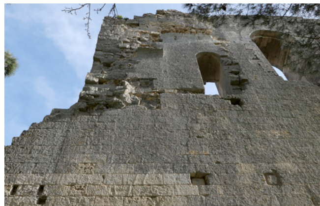
Figure 9. Gravina, castle's Palas , exterior part of north side with the remains of the toilet and traces of attachment indicating the position of the lost tower (Kappel 2023).
