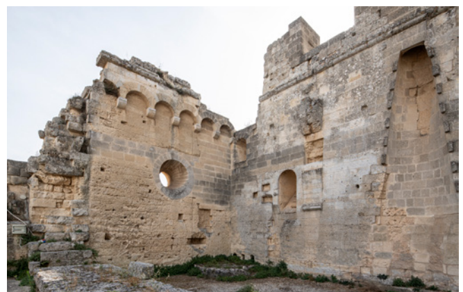
Figure 8. Gravina, castle's Palas , view of the reconstructed southwest corner and chimney, at the left the arch starter of GF 12 (Brandl 2023).
