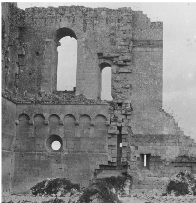
Figure 10. Gravina, castle's Palas, interior part of north side with a walled up breach in the lower section, detail, November 1905 (Kunsthistorisches Institut of Christian-Albrechts-Universität zu Kiel, Arthur Haseloffs Nachlässe, F 256).
