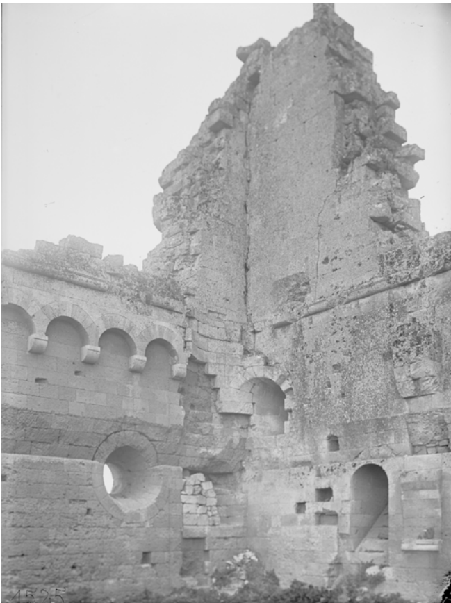
Figure 6. Gravina, castle's Palas , view of the inner corner of GF 19 with the remains of the spiral staircase and windows, October 1906 (Kunsthistorisches Institut of Christian-Albrechts-Universität zu Kiel, Arthur Haseloffs Nachlässe, PL 1525).
